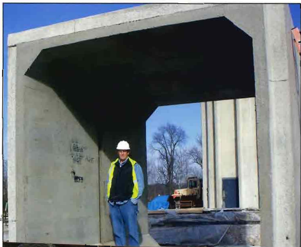
Burr Stanley, project manager - Bridge Division, stands in a newly cast box culvert. Delivery, which requires special accommodation due to the 10-foot height of the box culverts, will occur in the Spring and Summer of 2010.
